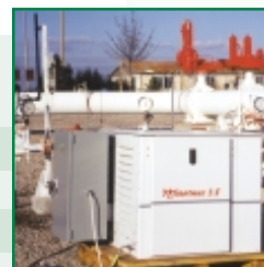
Remote Gasline Gate Valve Operation – Turkey
